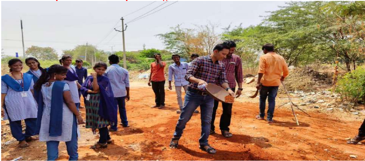
NSS VOLUNTERS AT ROAD REPAIR
