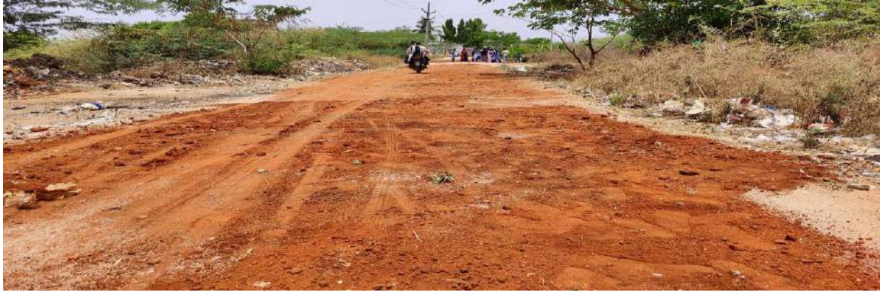
NSS Road Repair Work at adopted village
